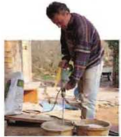
el albañil construction worker
