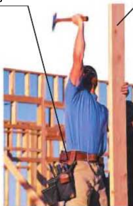
el albañil construction worker
